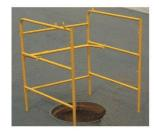
Once the cover has been lifted the area should be isolated using a suitable barrier system and signs, if the cover is hinged a wedge or break should be installed to prevent accidental closing and when the cover is replaced ensure it is seated properly and does not present a trip hazard.
