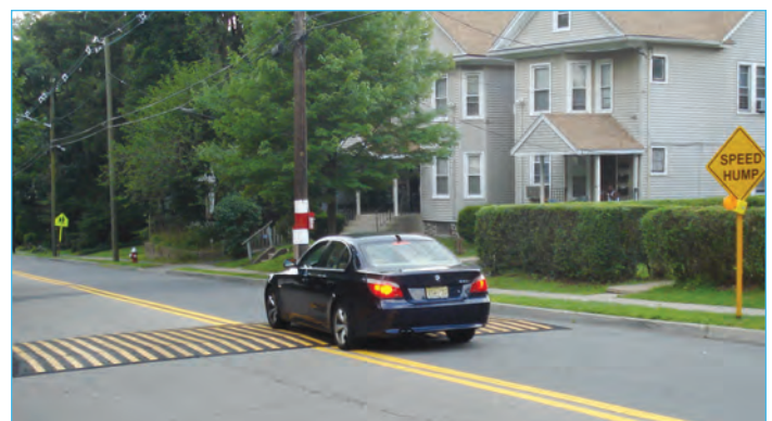
Speed Tables reduce pedestrian accidents by an average of 45%. Portable speed cushions are especially easy to install.
