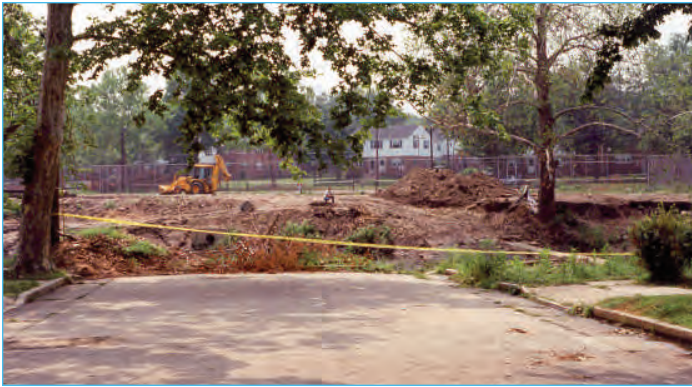
A classic traffic hazard – a dead-end street without a barrier where the road ends at a stream.
