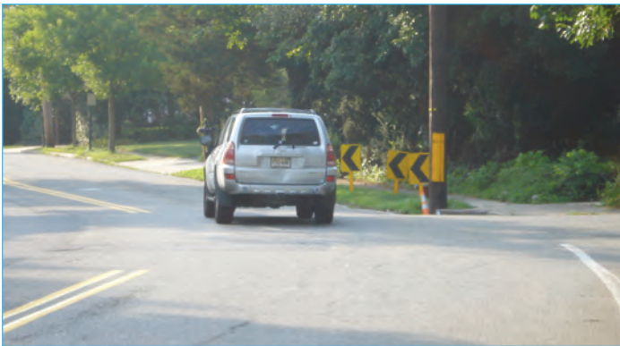
Curves need to be adequately marked.
