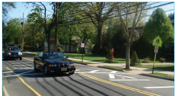
A raised crossing station was installed to slow traffic and to discourage children from crossing away from the guard.
