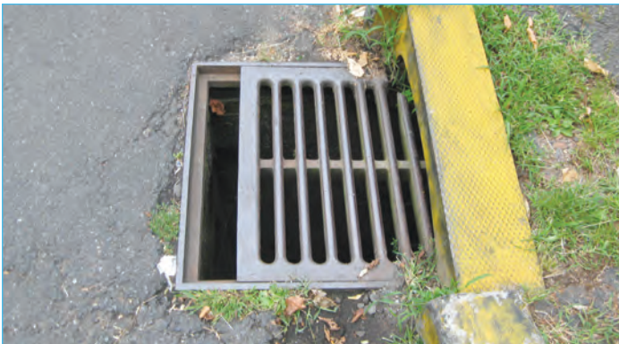
Pot holes and broken drainage grates present significant hazards to bicyclists, motorists and pedestrians.
